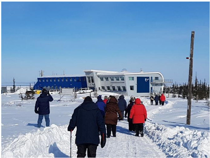
CNSC building, with tour group.
