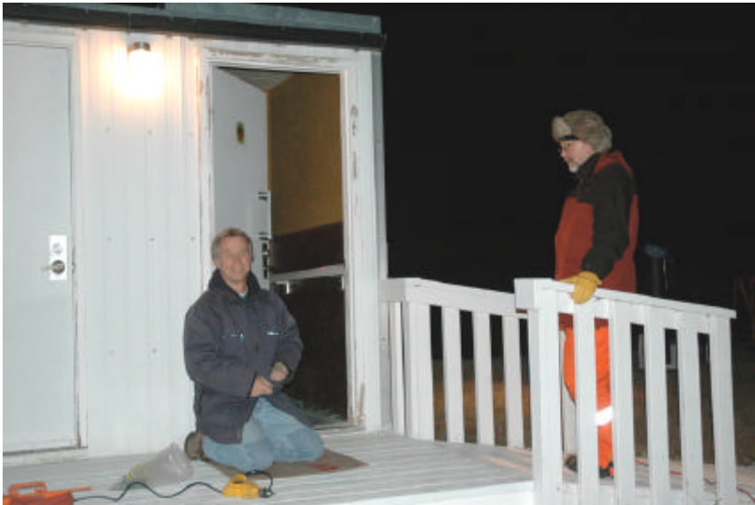
Darrell beams amid new decking that impressed Sleaford Open House visitors
